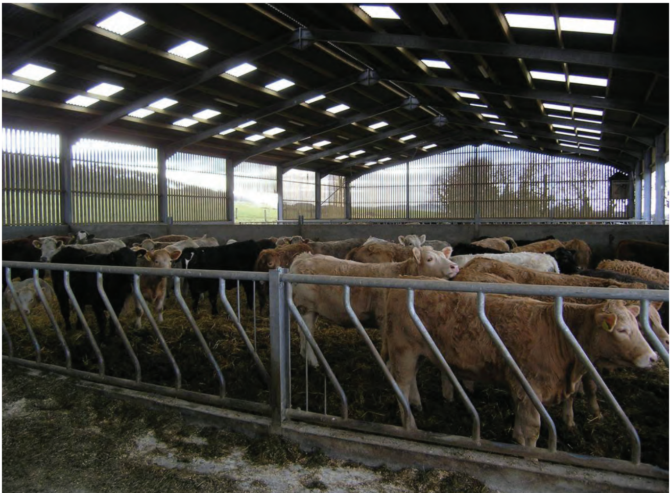
Good example of natural ventilation
